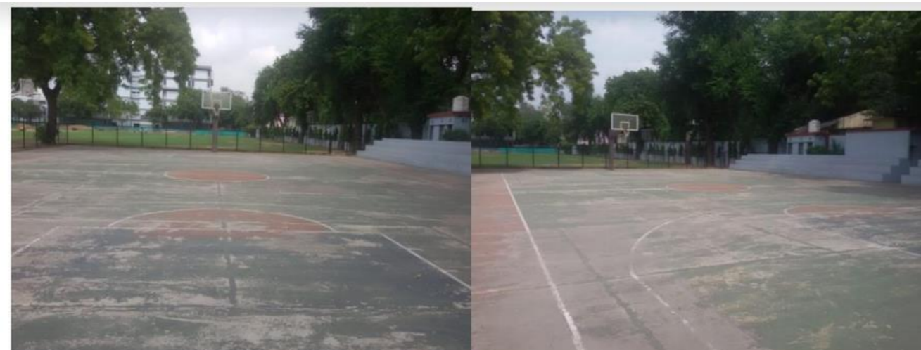
BASKETBALL COURTS (BEFORE)
